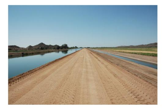
Fig. 2 Water supply canal (L) and drainage canal (R), Wellton-Mohawk irrigation and drainage district, Wellton, Arizona. [Note that these canals flow in opposite directions!].
