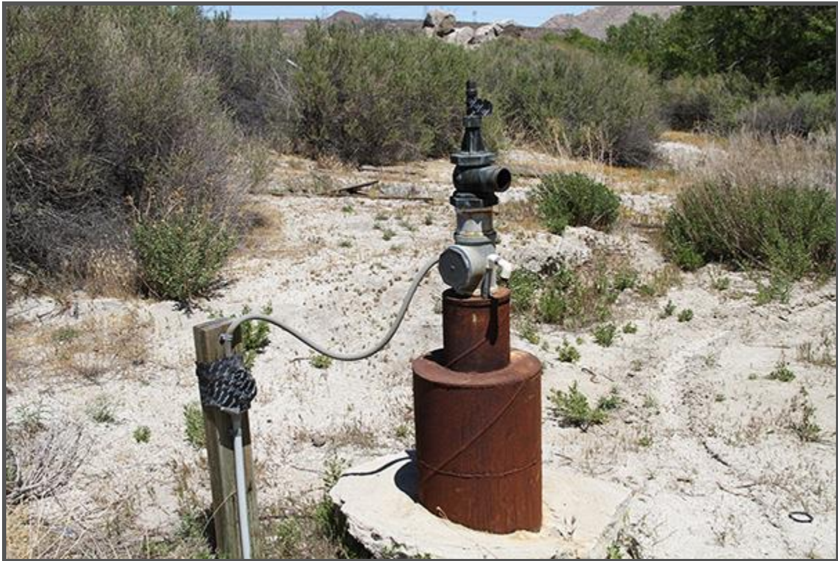
Fig. 33 Jacumba community well: Jacumba, San Diego County, California.
