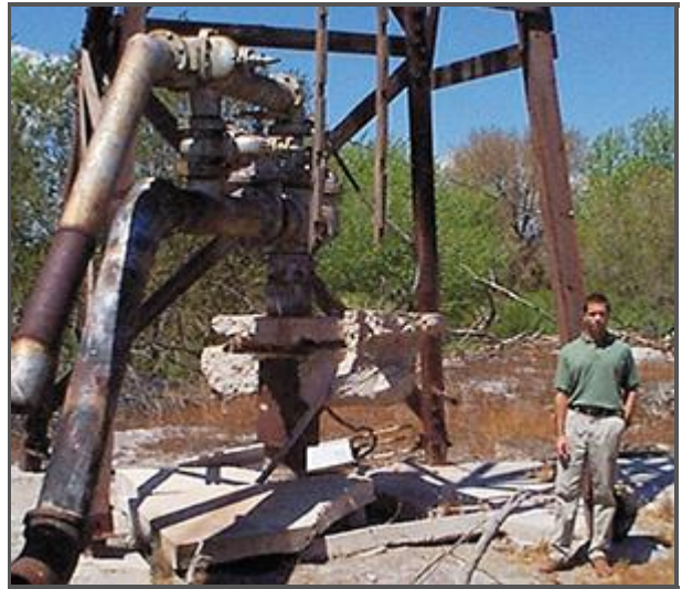
Fig. 28 Timed photographs of a protruding well in Las Vegas, Nevada, showing evidence of land subsidence (From Pavelko et al. : Las Vegas, Nevada, in U.S. Geological Survey Circular 1182).
