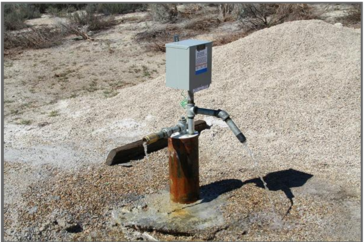
Fig. 48 New water well near Walker Creek, flowing under artesian conditions on September 18, 2013.
